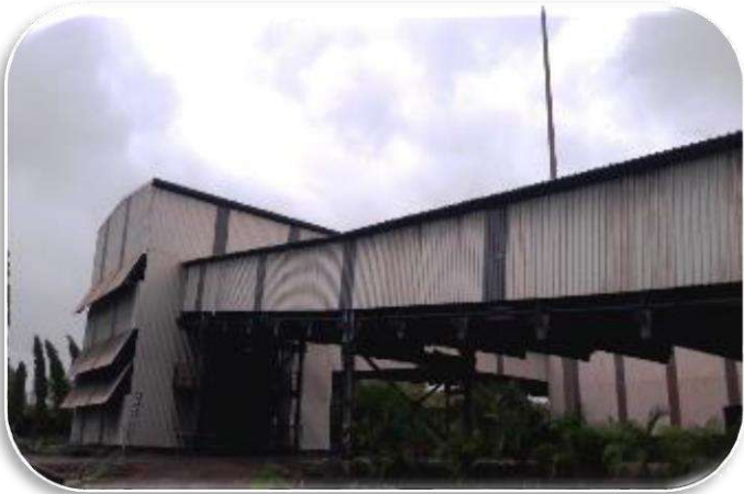
Covered Conveyor Belt
